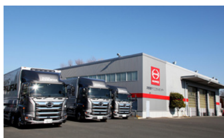
The Customer Technical Center
